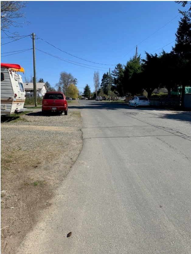
Figure 3 Frontage of 2219 and 2221 Dalton Road, looking south.
