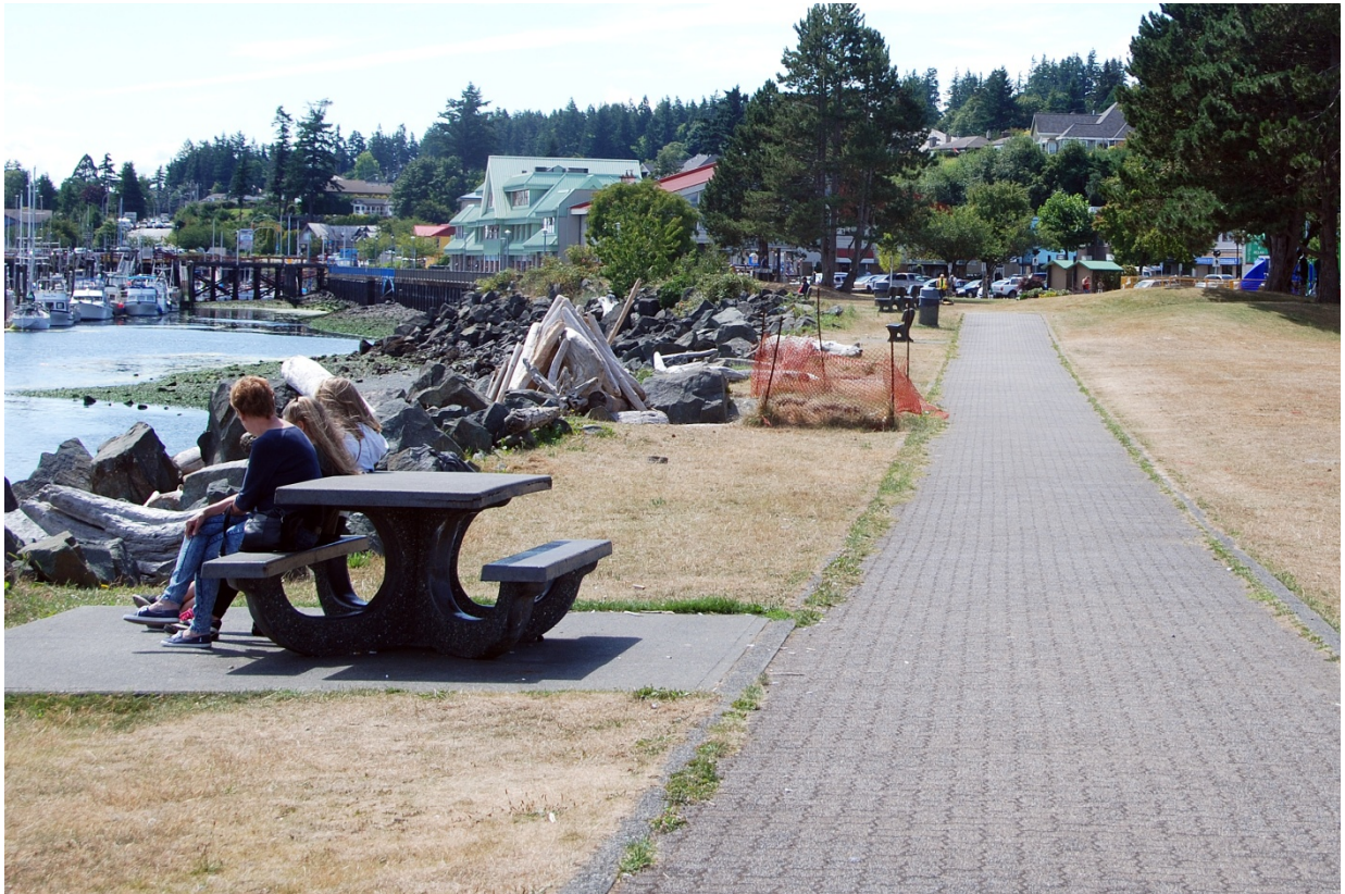
Figure 5.3 - Site furnishings require oversize concrete pads These features effectively require 3-4m of level land at the back of the beach. In the current armoured-bank situation, some of the slabs (and benches) have been damaged by over-topping waves (red snow fence - mid-ground). A few of the benches have been damaged by hurled logs during storms. Some of the site furnishings do not have pads extending fully back to the walkway limiting accessibility of the mobility-challenged.
