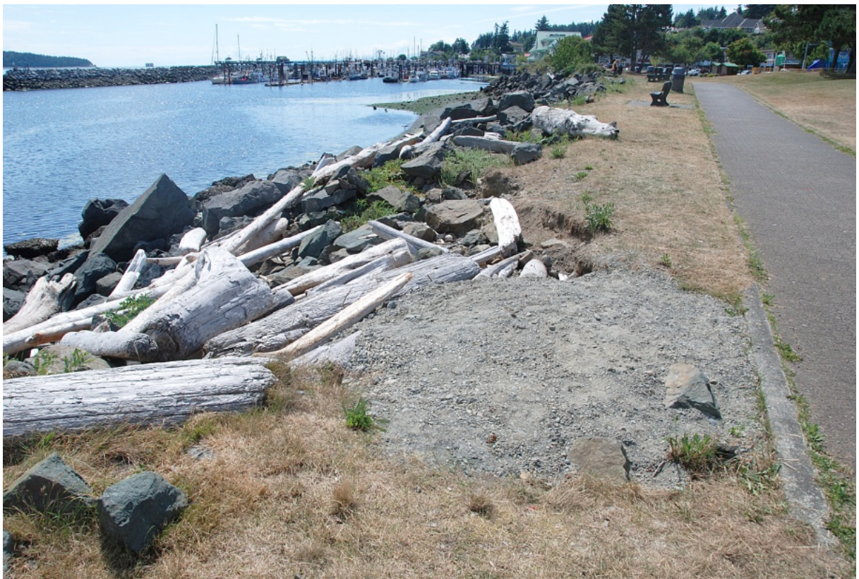
Figure 5.1: Seaward grass strip between walkway and rip-rap bank is subject to storm wave erosion.
