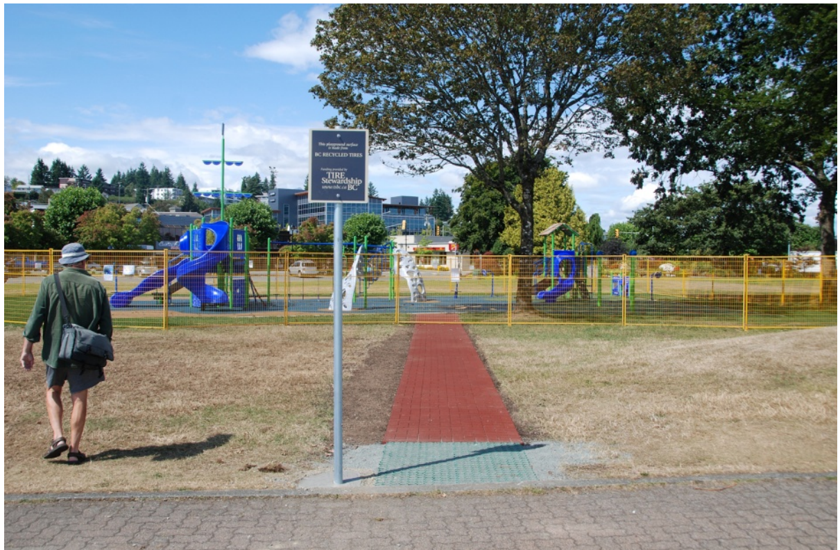
Figure 5.6: New Play Area constructed June-July 2016
