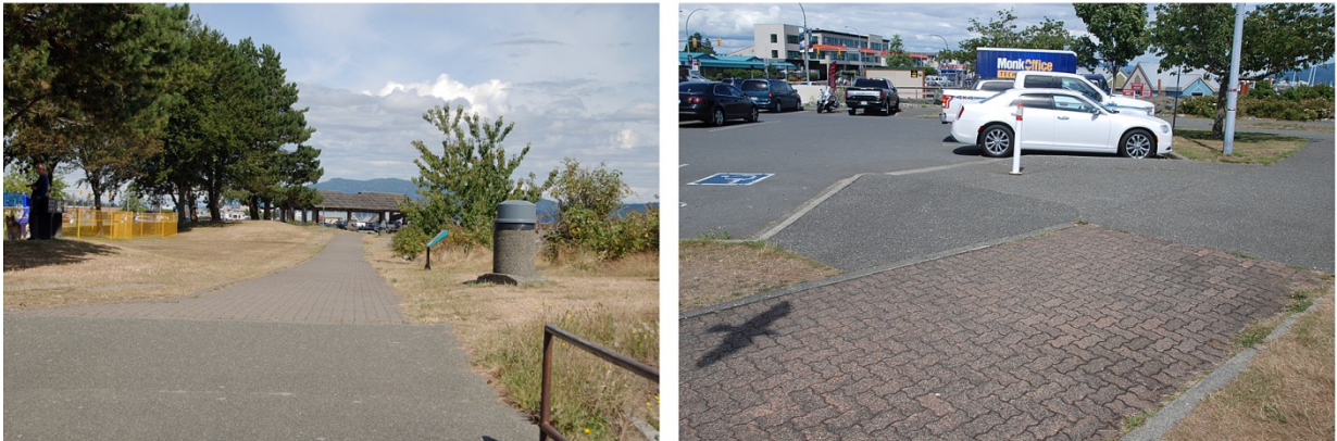
Figure 5.2 - Connections with adjacent walkways Sea Gull Walk (left) and at parking lot to north (right). Note abrupt grading transition at end of Sea Gull walk and difference in width. Sea Gull walk is elevated over an armoured shoreline and is therefore 'fixed'. Both walkways are exposed aggregate cast-in-place concrete. Current DFO policy does not support exposed aggregate finishing at the shoreline due to deleterious effects of washing off the surface retardant chemicals to fish habitat.
