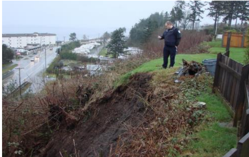
Surficial landslide, Murphy Street from the crest of slope to the Island Hwy, January 2020. The slide initiated in an area with 30+ years of historic yard waste dumping during a period of heavy rain.
