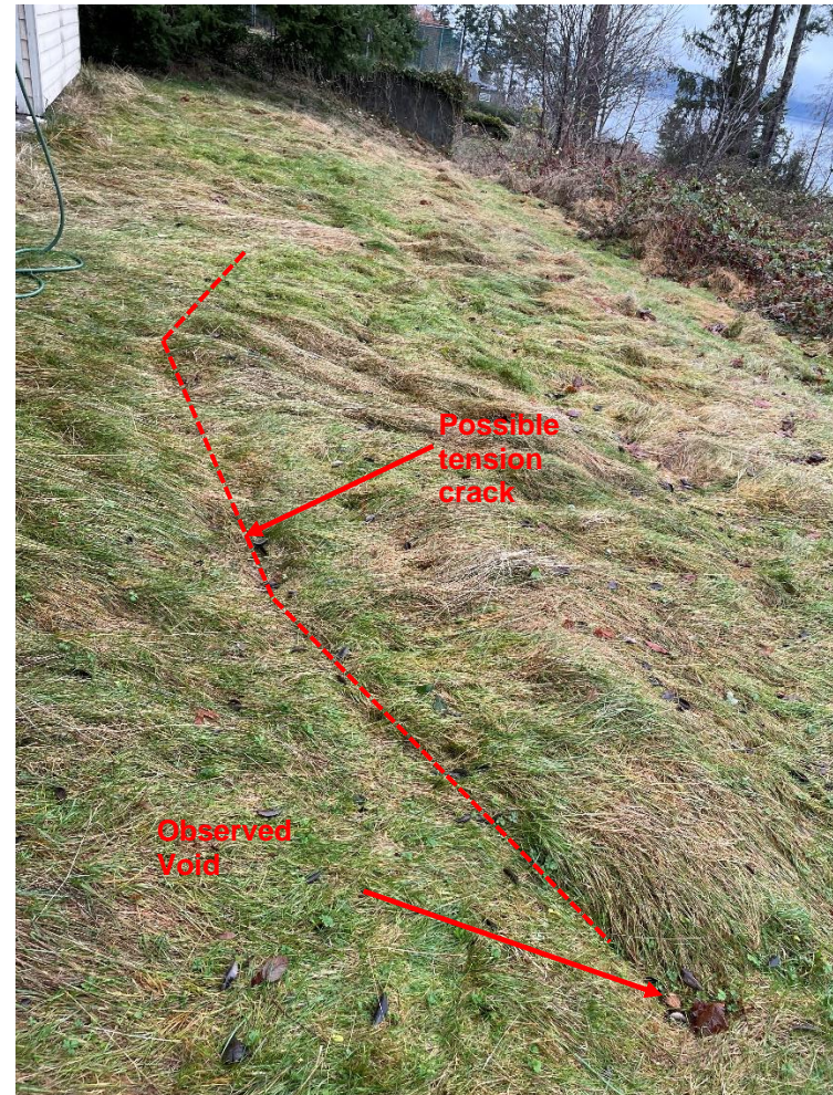
Photo 12: Grass covered backyard at 739 Ash Street. Possible tension crack visible in the grass area and void. City sewer line located between the visible crack and the crown of the landslide.
