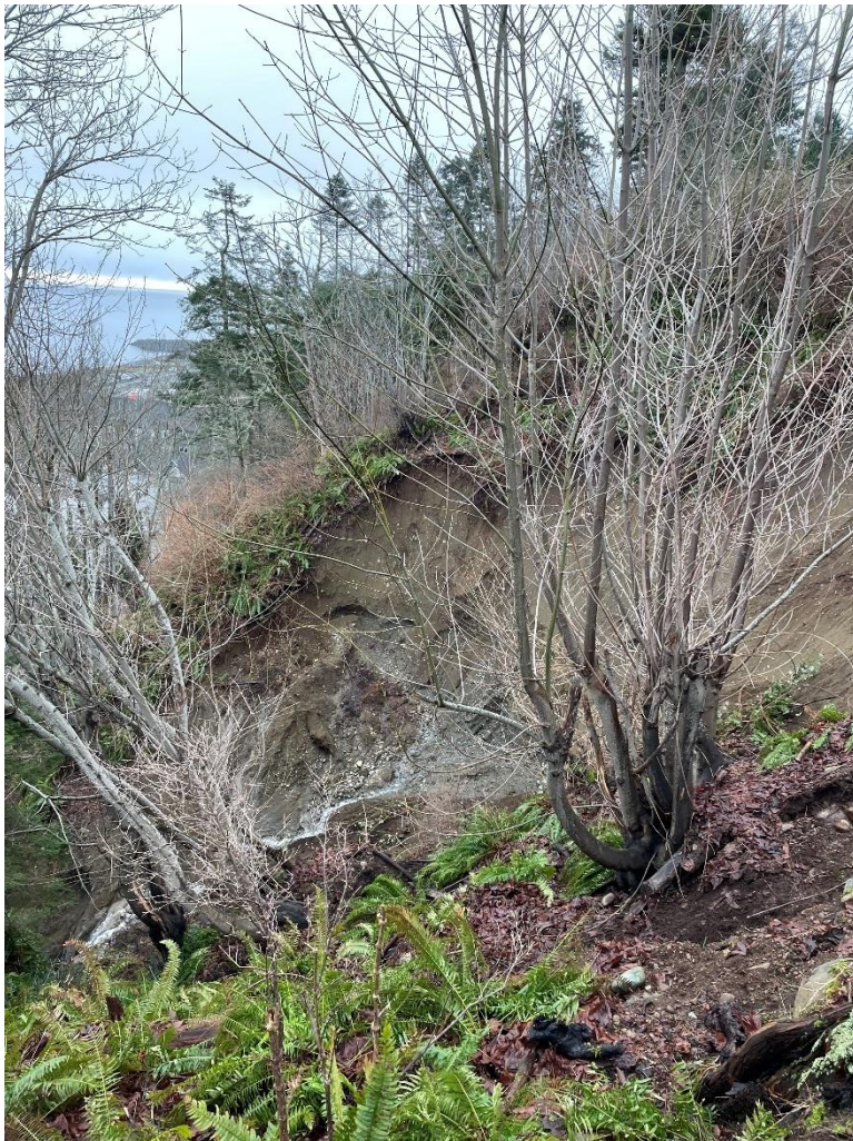
Photo 11: Probable natural spring emanating from the southern face of the failure surface.
