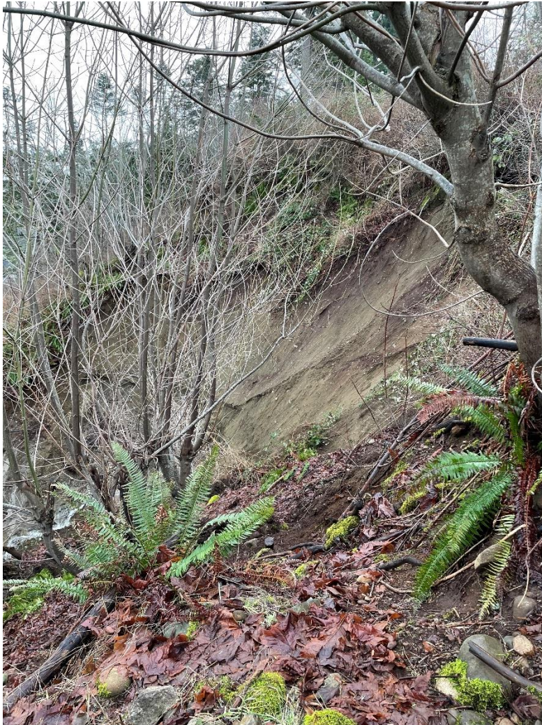
Photo 9 : View of the head scarp from the north.
