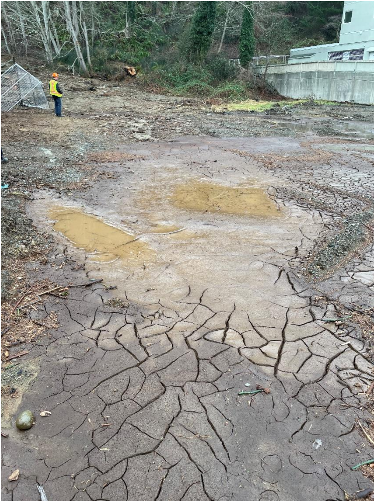
Photo 1 : 738 South Island Hwy, mudslide deposit at toe of failed slope.
