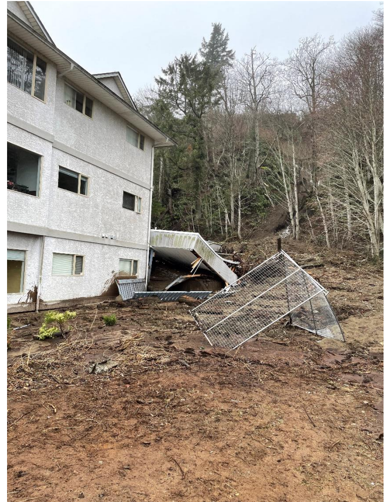
Photo 2: 738 South Island Hwy, damaged structure at toe of failed slope and soil debris from the landslide.
