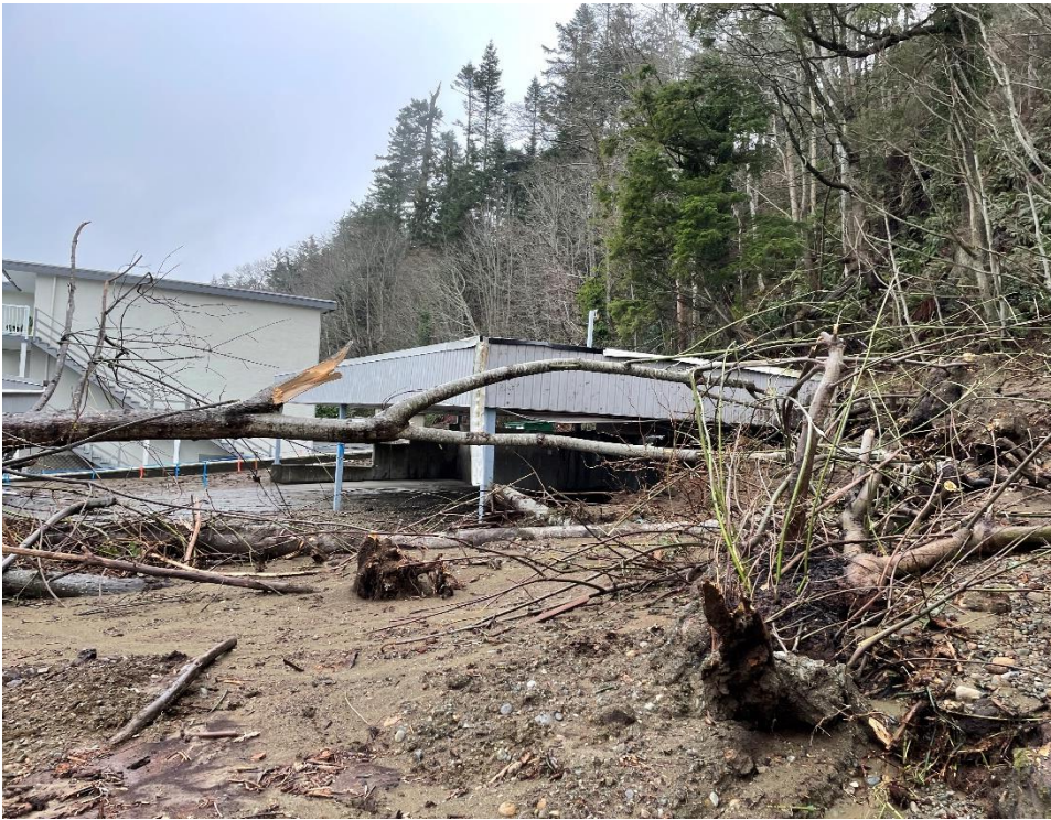
Photo 3 : 738 South Island Hwy, damaged structure and torn out trees at toe of failed slope.
