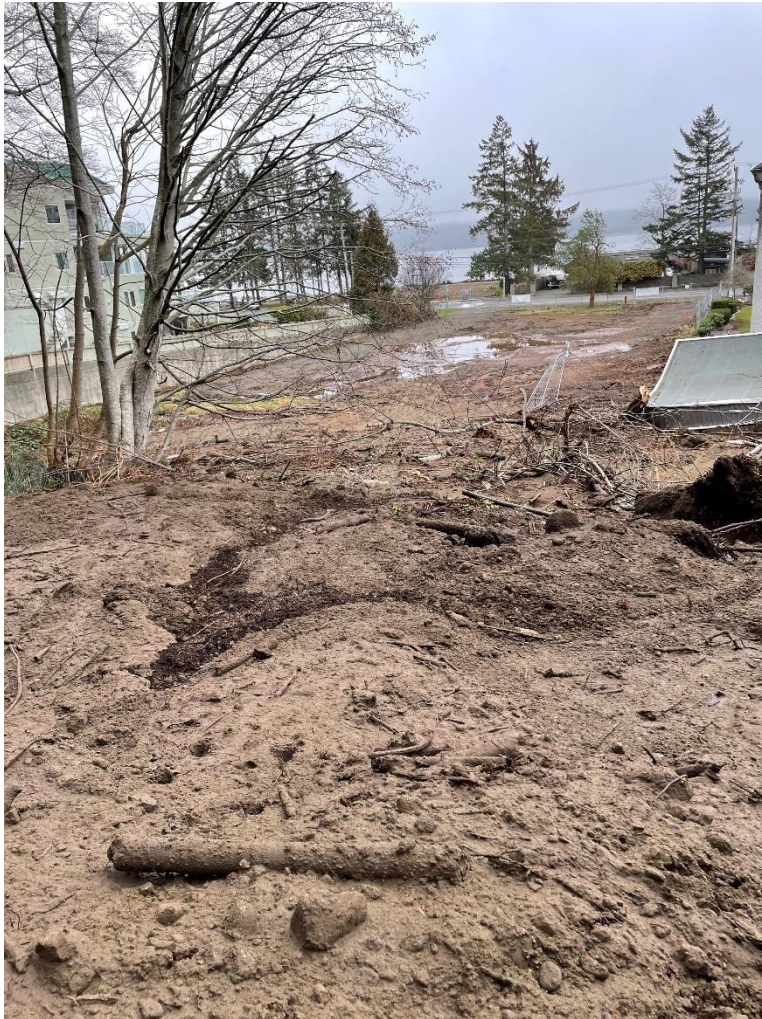
Photo 7: Debris at toe of failed slope.
