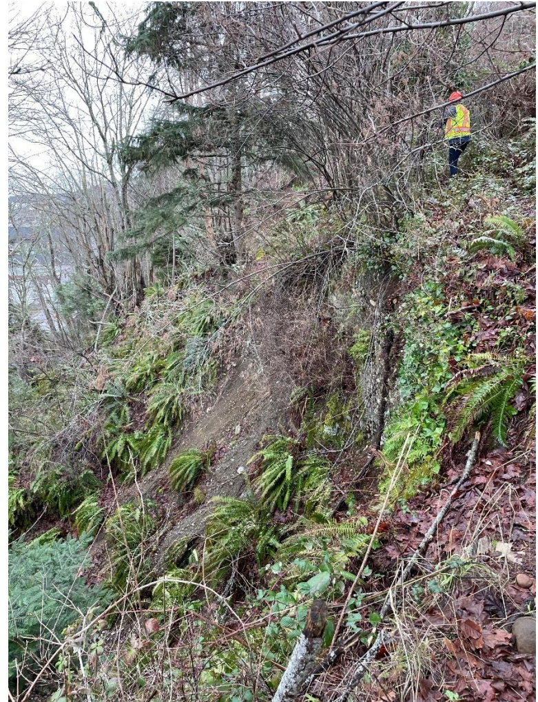
Photo 8: Shallow slope failure in the slope on property 723 Ash Street, north of the assessed failed slope.
