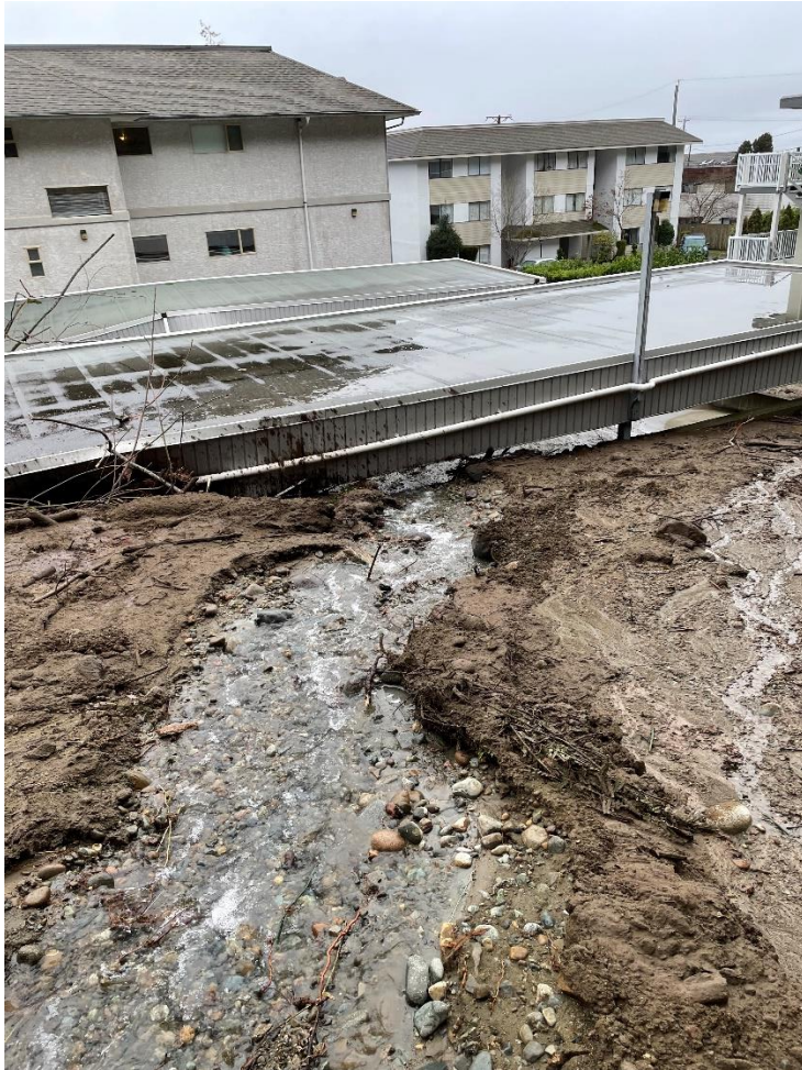
Photo 5 : Water flow towards 738 South Island Hwy Building.
