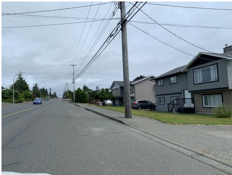
Examples of obstructed sidewalks
