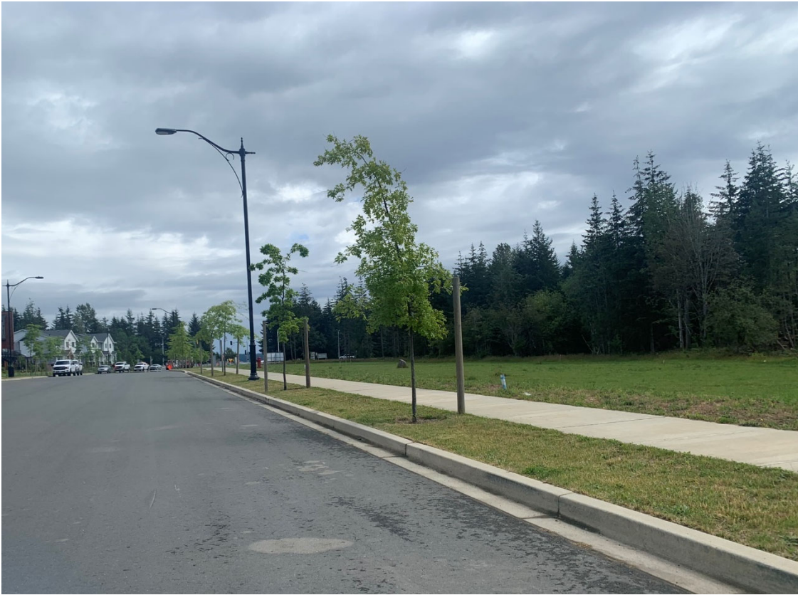
This section of S Alder Street is an example of where a separated sidewalk facility is available for people walking / rolling.
