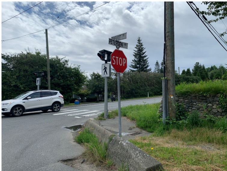
Example of an inaccessible crosswalk and curb ramp at the intersection of Cheviot Road and Petersen Road (left) and a double curb ramp design (right) from the BC Active Transportation Design Guide.
