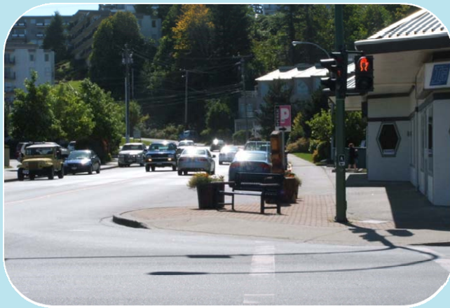
Below: Curb bulge at Cedar Street and 11th Avenue requires increased driver attention for turns.
