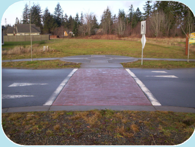
Above: Raised crosswalk with textured pattern on Maryland Road reminds drivers to drive with care.
