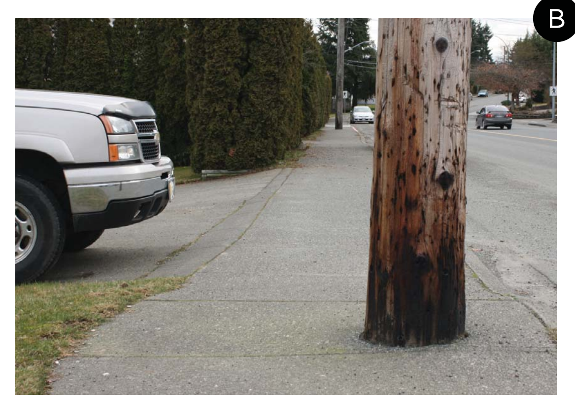
Utility poles in the middle of the sidewalk make sidewalks uncomfortable for groups of pedestrians and unpassable for wheelchairs and most other mobility devices.
