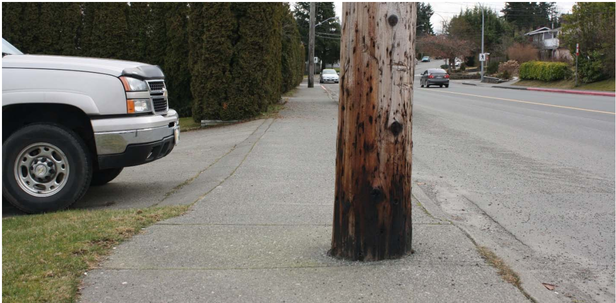
An example of a utility pole in the sidewalk which reduces the functional width of the sidewalk and makes inaccessible for wheelchairs and other mobility devices
