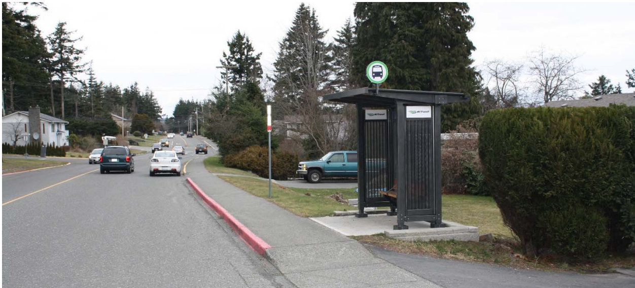
Recent bus stop installations at Coronation Park and Evergreen Road (above) should be used as examples for future bus stop improvements
