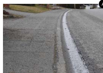
Sidewalks with "mountable" curbs do not provide a barrier between pedestrians and vehicles and may result in vehicles parked on the sidewalk.
