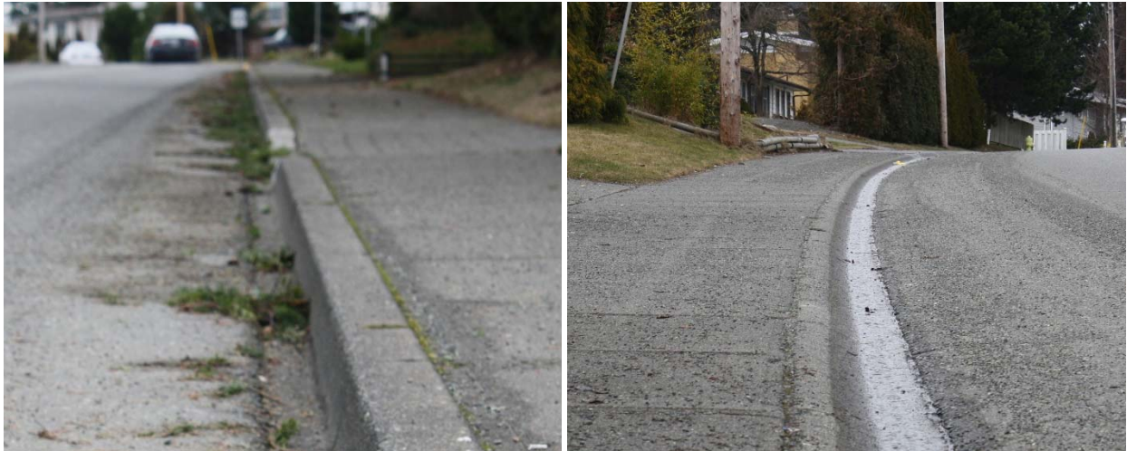
A barrier curb (left) provides a physical barrier between the sidewalk and roadway, while a mountable curb (right) permits vehicles to mount the sidewalk.
