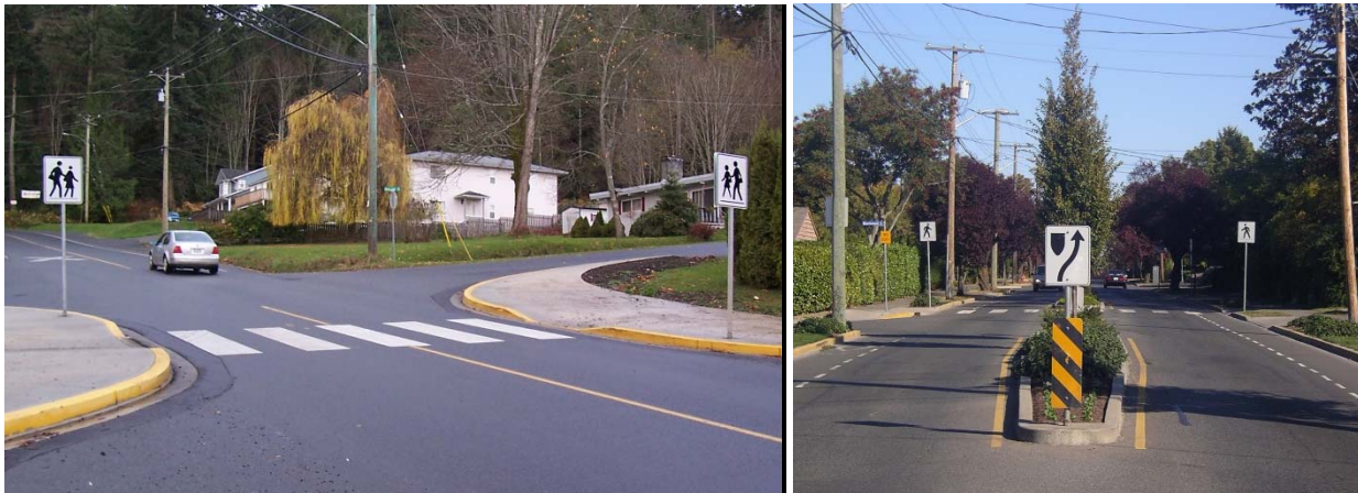
Curb extensions (left) and raised median islands (right) will be used along Alder Street to enhance pedestrian crossings and manage vehicle speeds.
