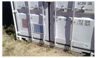
Suggested solutions include a lower ventilation opening in the lower door (above) and an upper ventilation opening and wind vent (below). Photos courtesy of BC Hydro Fire Marshal's office.
