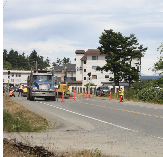
Crews preparing the highway/laydown area for work this summer.
