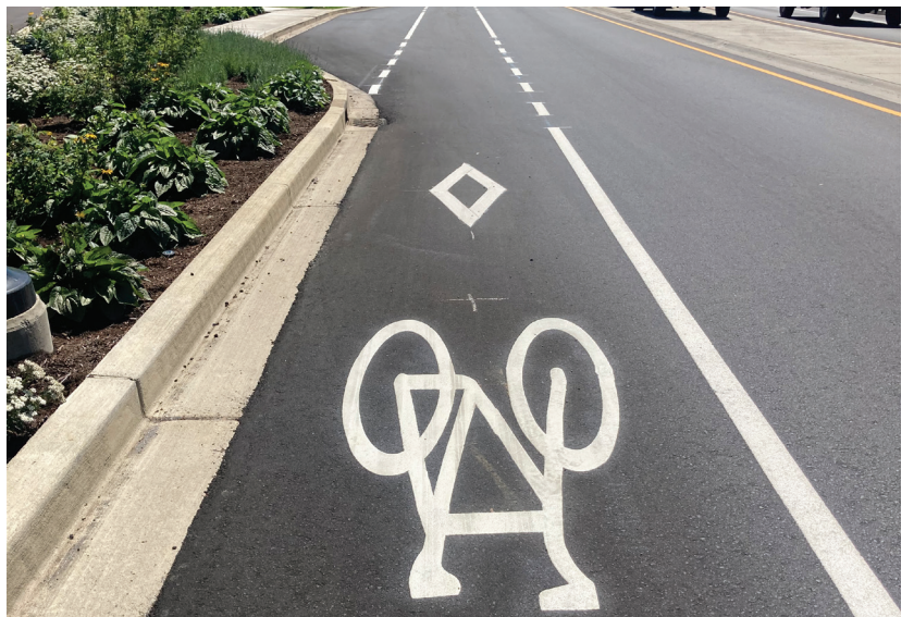
SMOOTH RIDE: Final paving gives the area a polished look while providing dedicated bicycle lanes.
