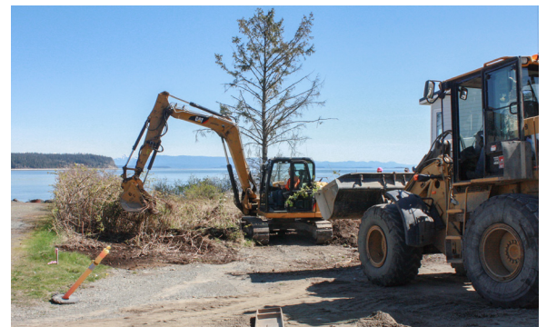
A new parklet/beach access is being installed on an unused road right of way
