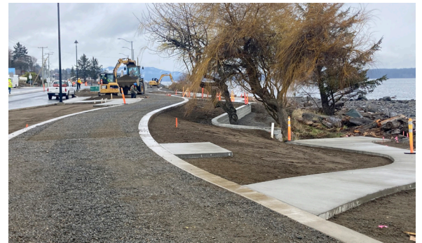
Crews work to prepare the new Ellis Park for planting and walkway paving
