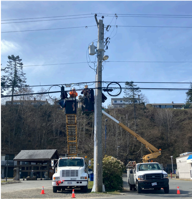
Crews are working to move the overhead services underground
