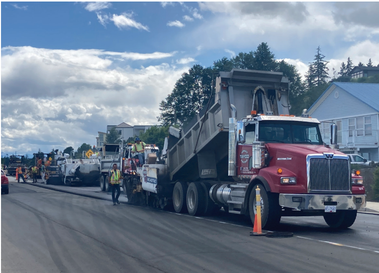
Final paving being completed along the highway.
