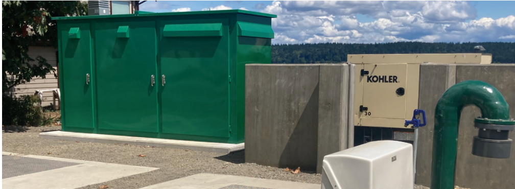
One of the two fully operational lift stations
