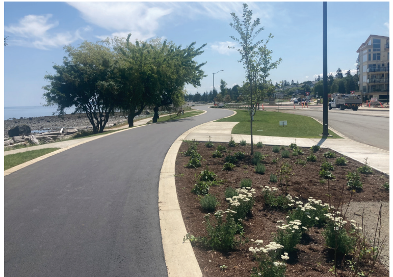
A fresh new look! Crews are working hard to finish up final landscaping and park installations that will complement the completed paving work.
