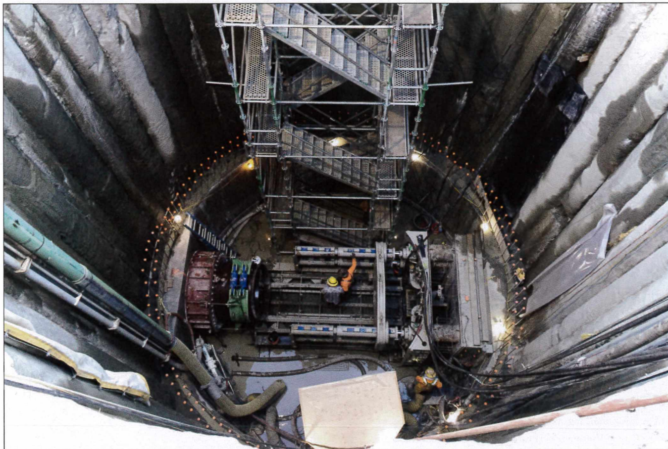
The John Hart Lake project's caisson intake structure for the pump station temporarily served as microtunneling jacking shaft.
