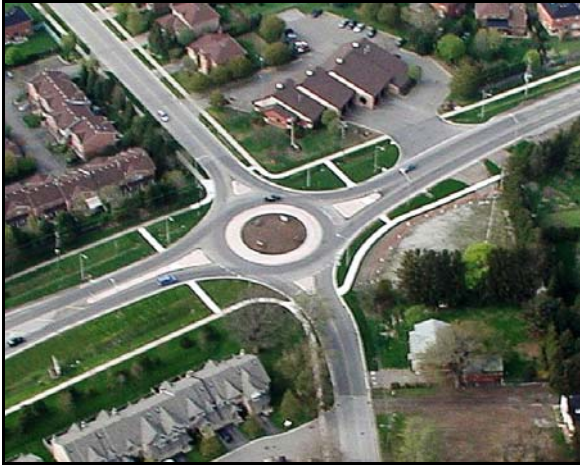
Figure 3 — Single-lane roundabout, Hamilton ON
