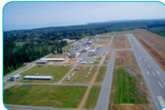
Airport Runway Extension Project - before
