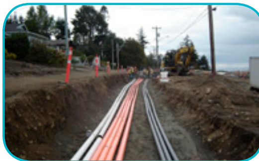
Highway 19A - during construction
