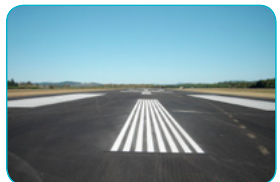
Airport Runway Extension Project - after
