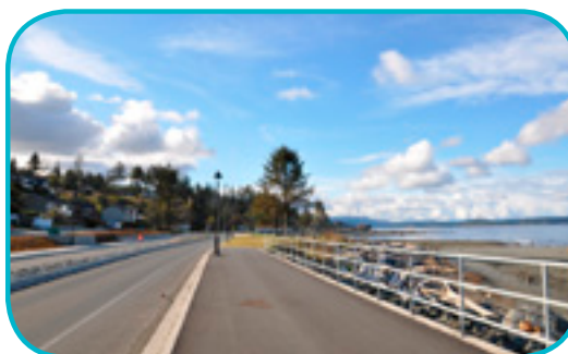
Highway 19A - after construction
